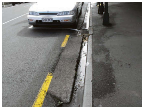
Gutters pose a problem when crossing the road.
